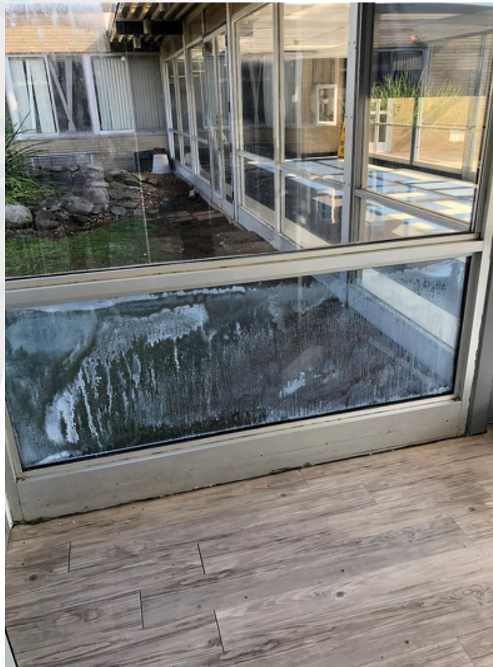
Existing Middle School Building Conditions
