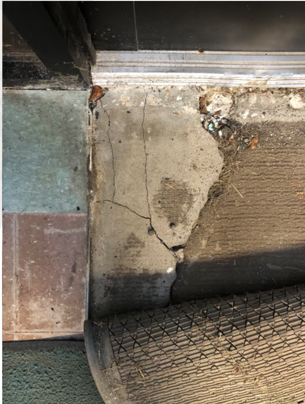
Existing Middle School Building Conditions
